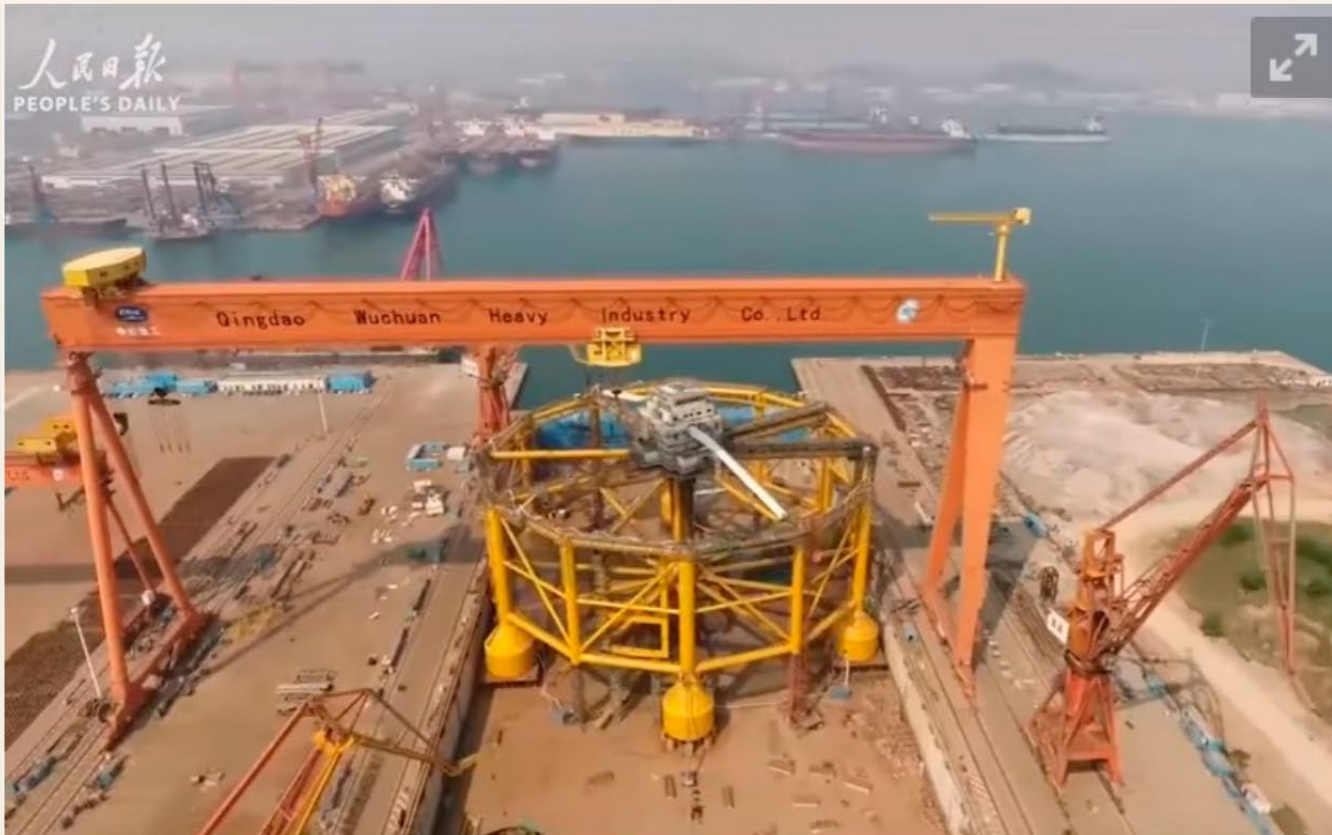
SalMar's Ocean Farm 1 under construction in Qingdao, China. Credit: People's Daily
