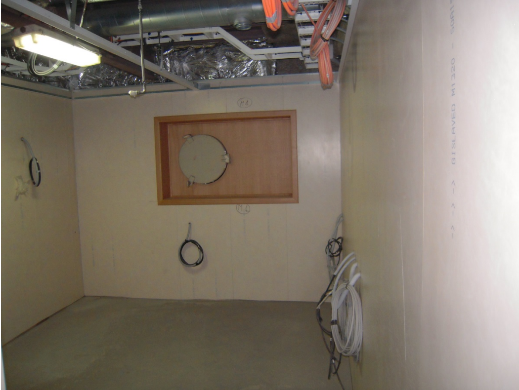
Cabins on Tween and Main deck ready for ceiling panel and floor cover.
