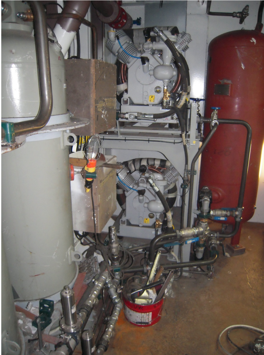
Pipe termination and assembly of auxiliary components progressing
