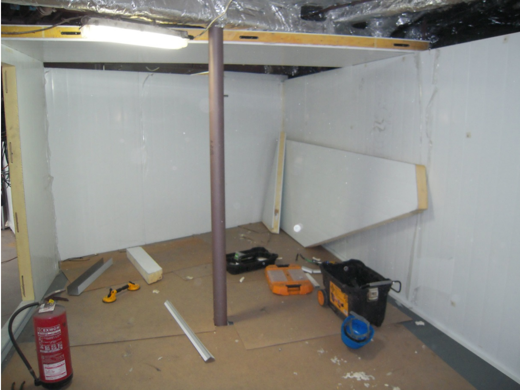
Freezer rooms in progress
