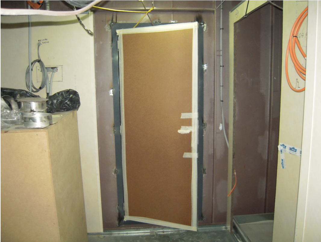
A-door installation in progress
