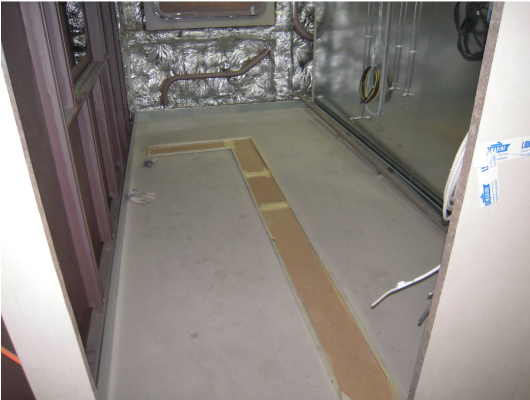
Pantry floor ready for tiling
