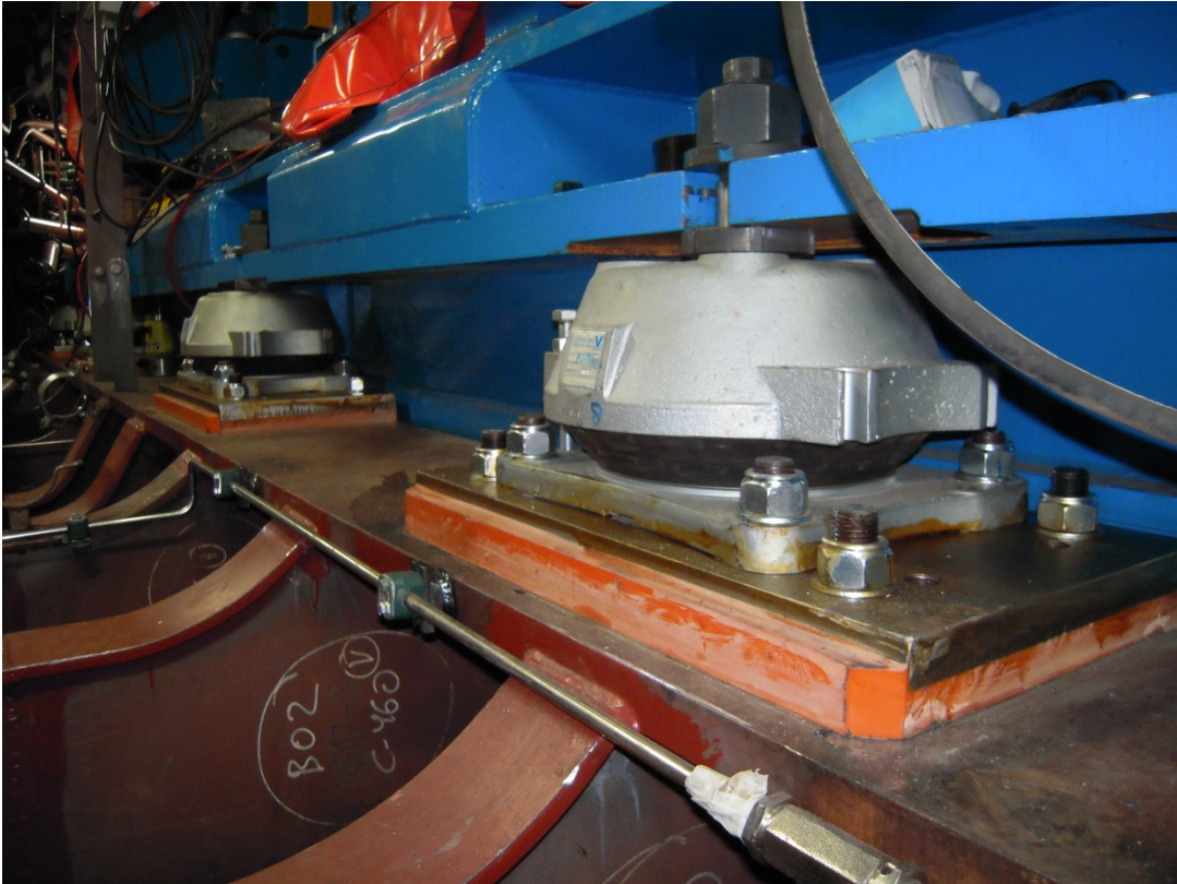
Propulsion motors aligned and chock fastened
